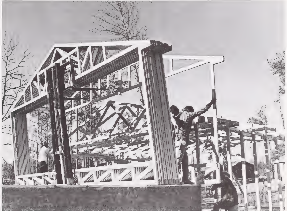
Using the Truss-Frame System, a small crew of laborers can frame up an average house in just a few hours.
